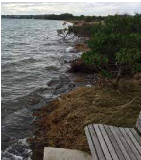
Bird roost compromised during a large tide. 04/02/2018.
