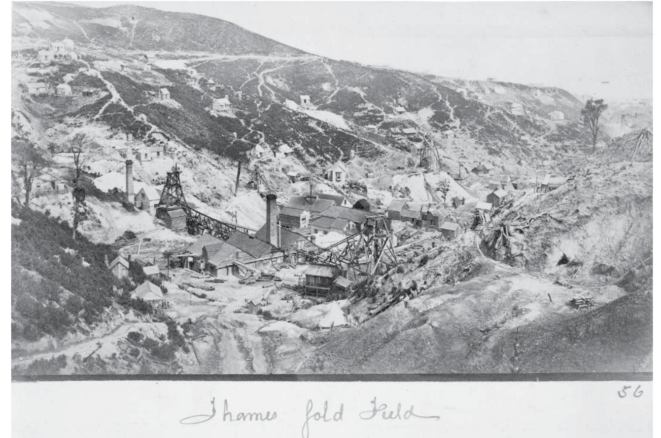
Gold mining batteries, Moanataiari Valley, Thames. © Sherring, W W: Photographs of gold mining near Thames and view of the Wairarapa Plains. Ref: PAColl-7395-1. Alexander Turnbull Library, Wellington, New Zealand. /records/23203728
