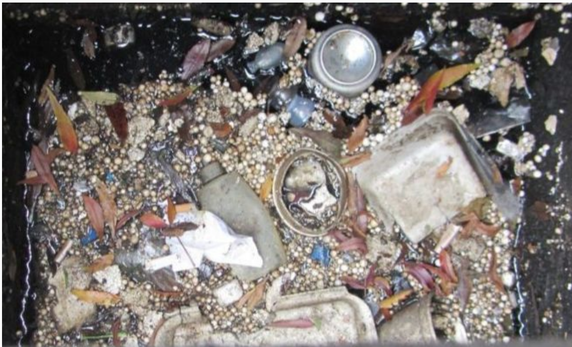
Catchpit in Line Rd with polystyrene beads and containers, Glen Innes. Photo credit: Beth Evans
